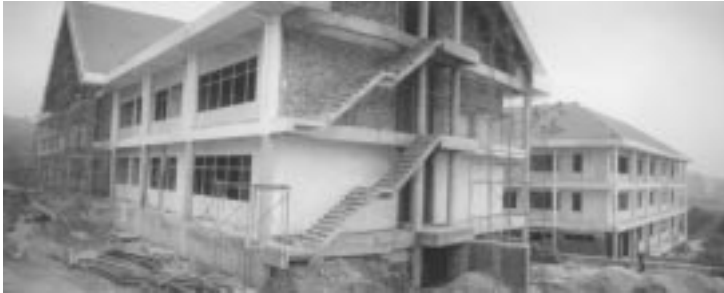
Figure 13 CEPP during construction (1996)
